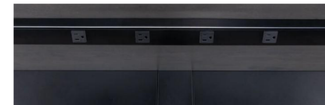
BLACK UNDER CABINET POWER STRIP (UNDER ALL UPPER CABINETS)
